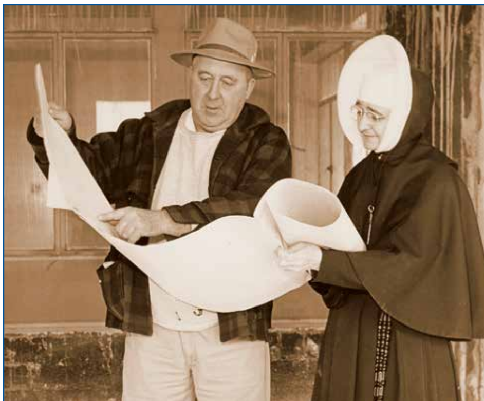
Sister Ernestine Marie Reisenauer, S.P., administrator, looking over plans with construction foreman Mike Kadera, Providence Hospital, Portland, Oregon, 1960s.
